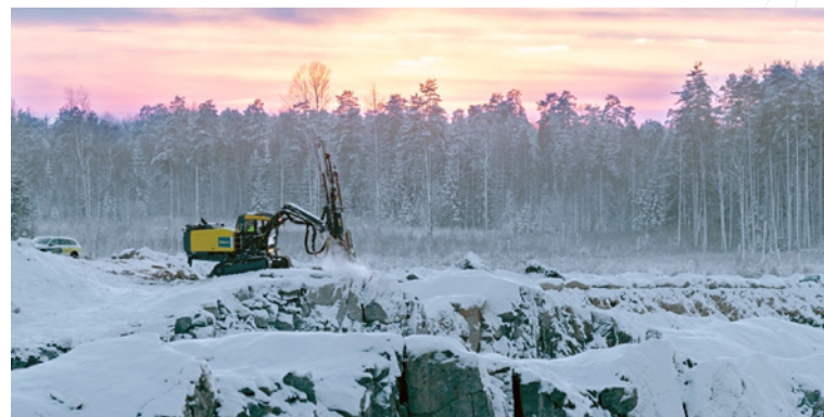
Drilling machine (Credit: EPIROC)
