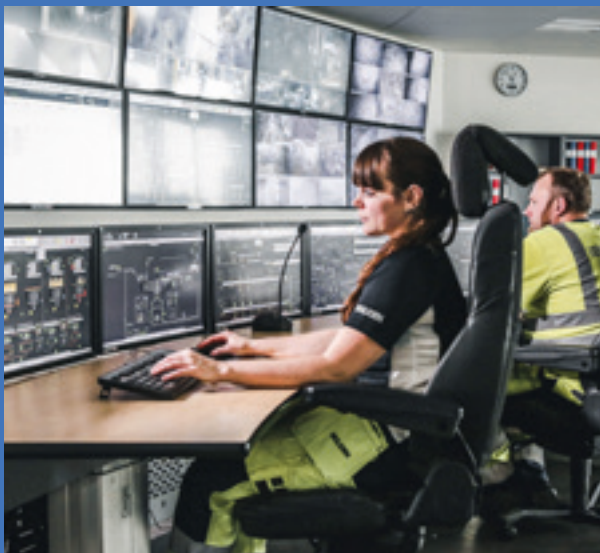
Control room, Garpenberg mine, Sweden (Credit: Boliden)
