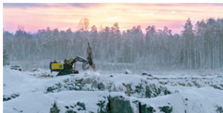
Drilling machine (Credit: EPIROC)
