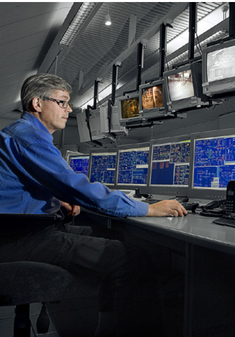
Boliden Harjavalta smelter control room. Picture provided courtesy of Boliden.
